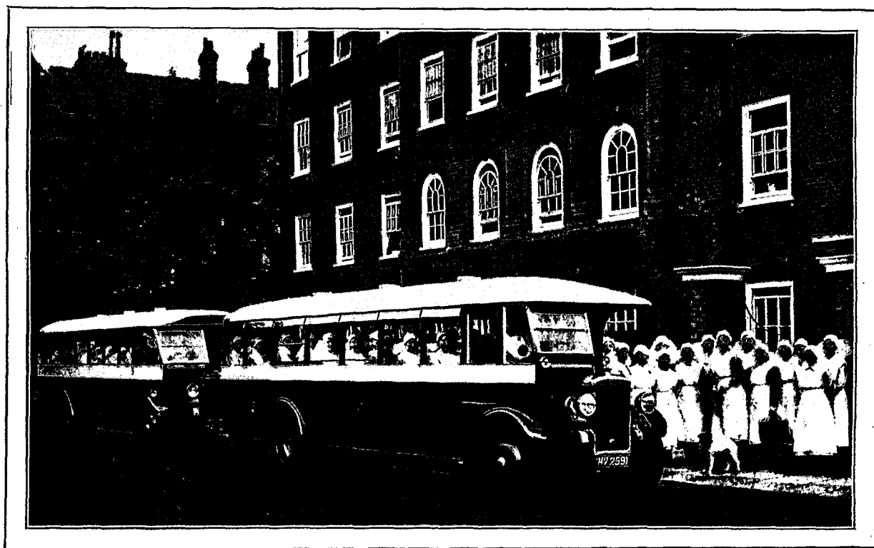
THE NEW NURSES' HOME, HAVERSTOCK HILL, N.W.3. Motor Coaches conveying the Nursing Staff to Charing Cross Hospital.
